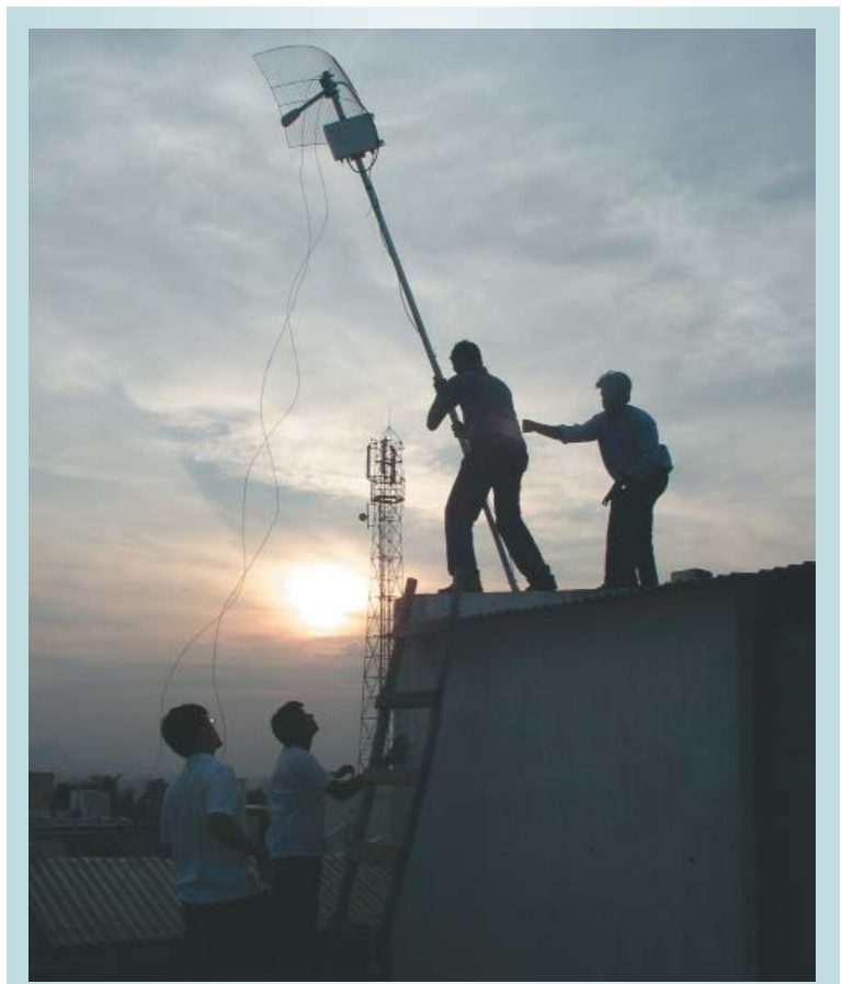
Figure 2. Students and village residents putting up a long-distance Wi-Fi link at sunset in southern India. Wireless technologies have the potential to provide a backbone that offers connectivity down to the village level.
